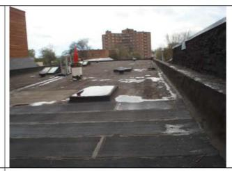
The field of the roof towards the front of the building has had modified bitumen roofing installed over the existing roof.
